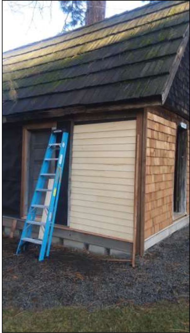
FIGURE 5. WEST SIDE DOORWAY, AND THE FIRST OF THE CLAPBOARDS GOING ON!
