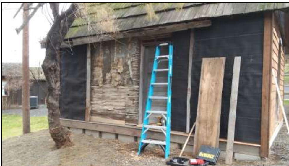
FIGURE 2. PUTTING TARPAPER ON THE WEST WALL.
