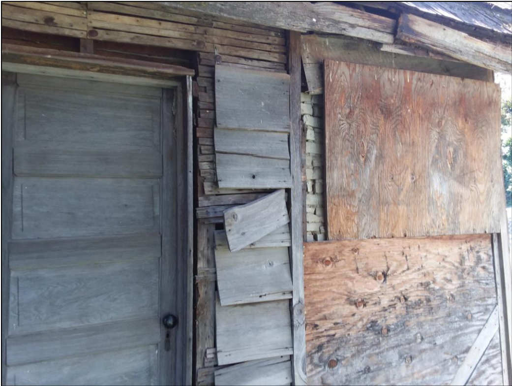
FIGURE 15: WESTERN EXTERIOR WALL SHOWING LATH, AND BRICK INFILLING.
