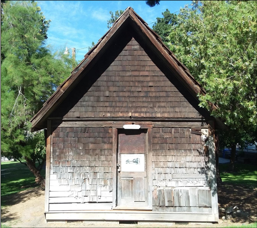
FIGURE 1: SOUTHERN WALL OF THE GARDENER'S COTTAGE AT FORT DALLES MUSEUM.
