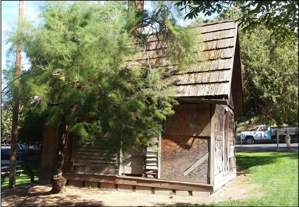
FIGURE 2: WESTERN WALL OF THE GARDENER'S COTTAGE, FORT DALLES MUSEUM.
