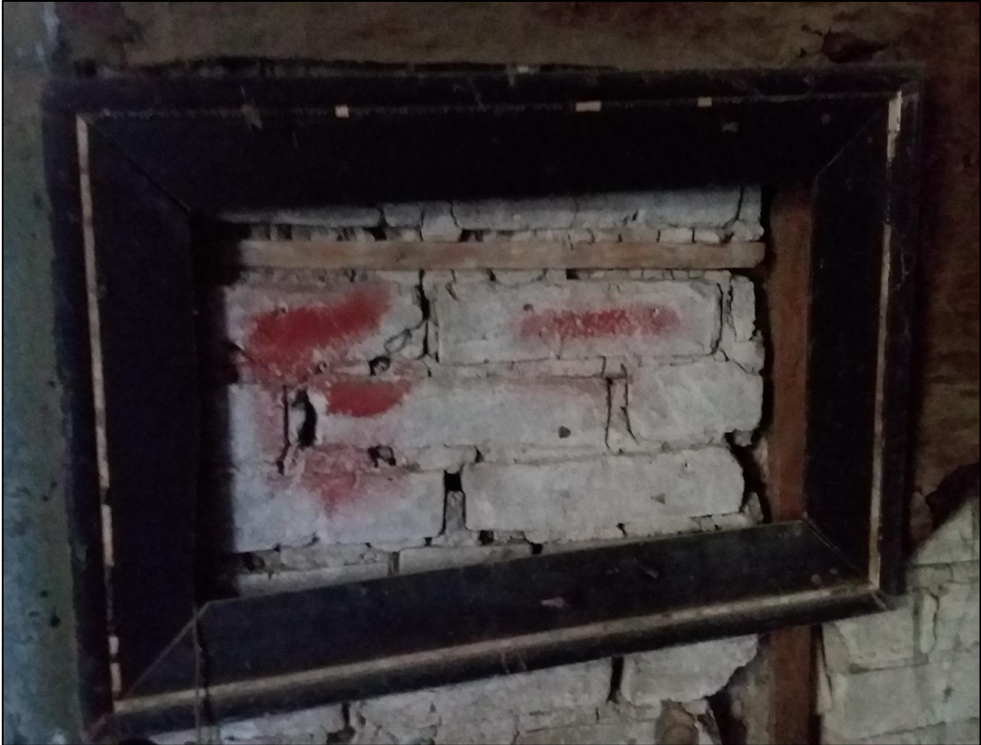
FIGURE 12: DISPLAY FRAME SHOWING BRICK INFILLING OF EXTERIOR WALLS.
