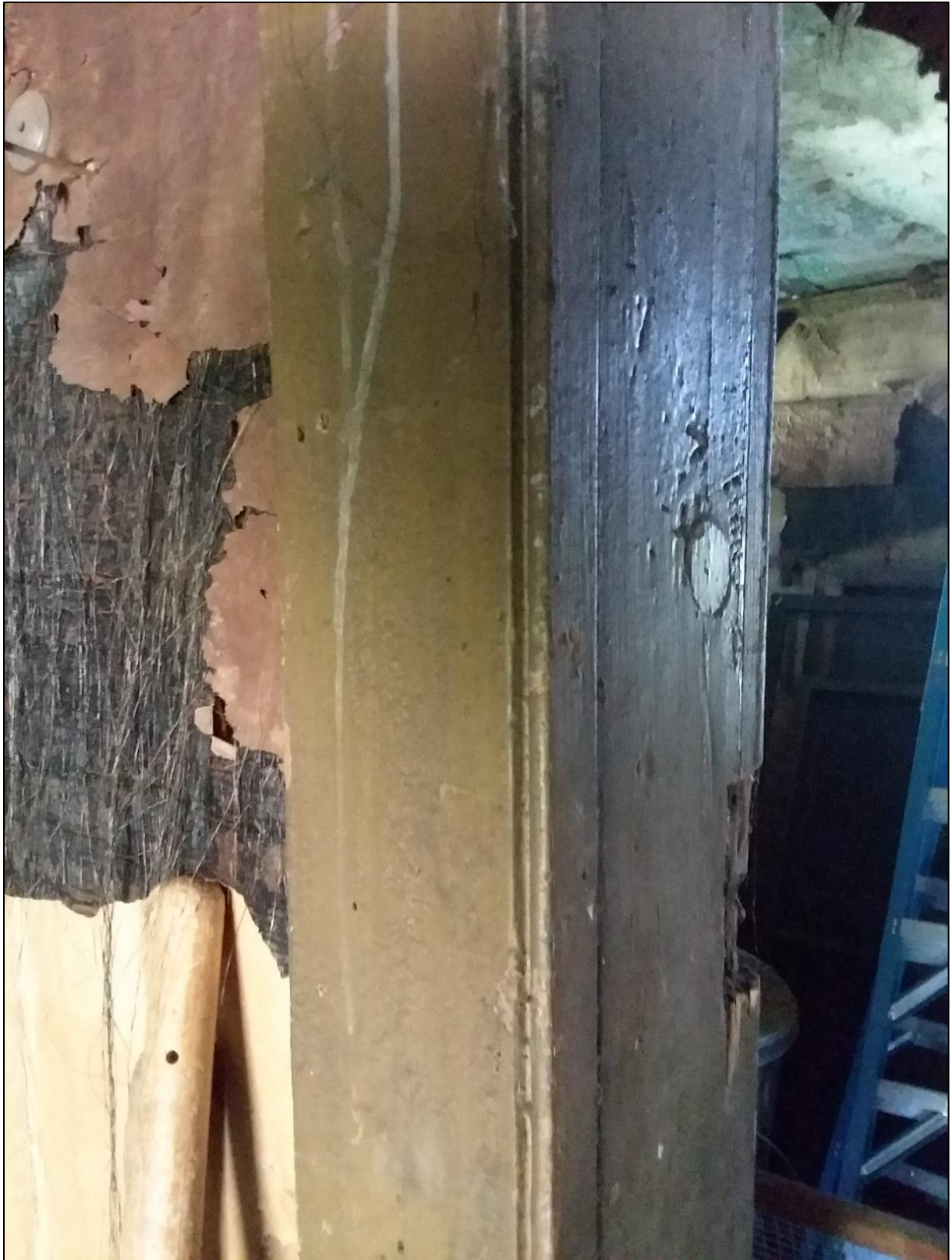
FIGURE 11: DETAIL OF TRIM AROUND INTERIOR DOORWAY, THE SAME MOLDING PATTERN AS IN THE 1856 SURGEON'S QUARTERS.
