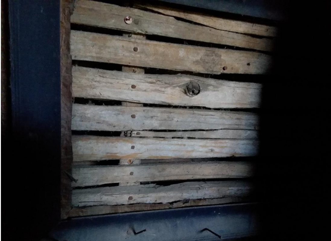
FIGURE 13: DISPLAY FRAME SHOWING HAND SPLIT LATH ON INTERIOR WALLS.
