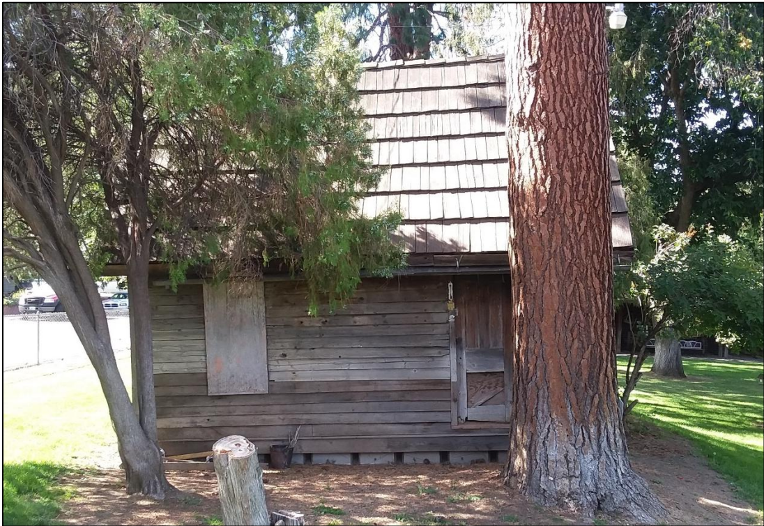
FIGURE 4: EASTERN WALL OF THE GARDENER'S COTTAGE, FORT DALLES MUSEUM.
