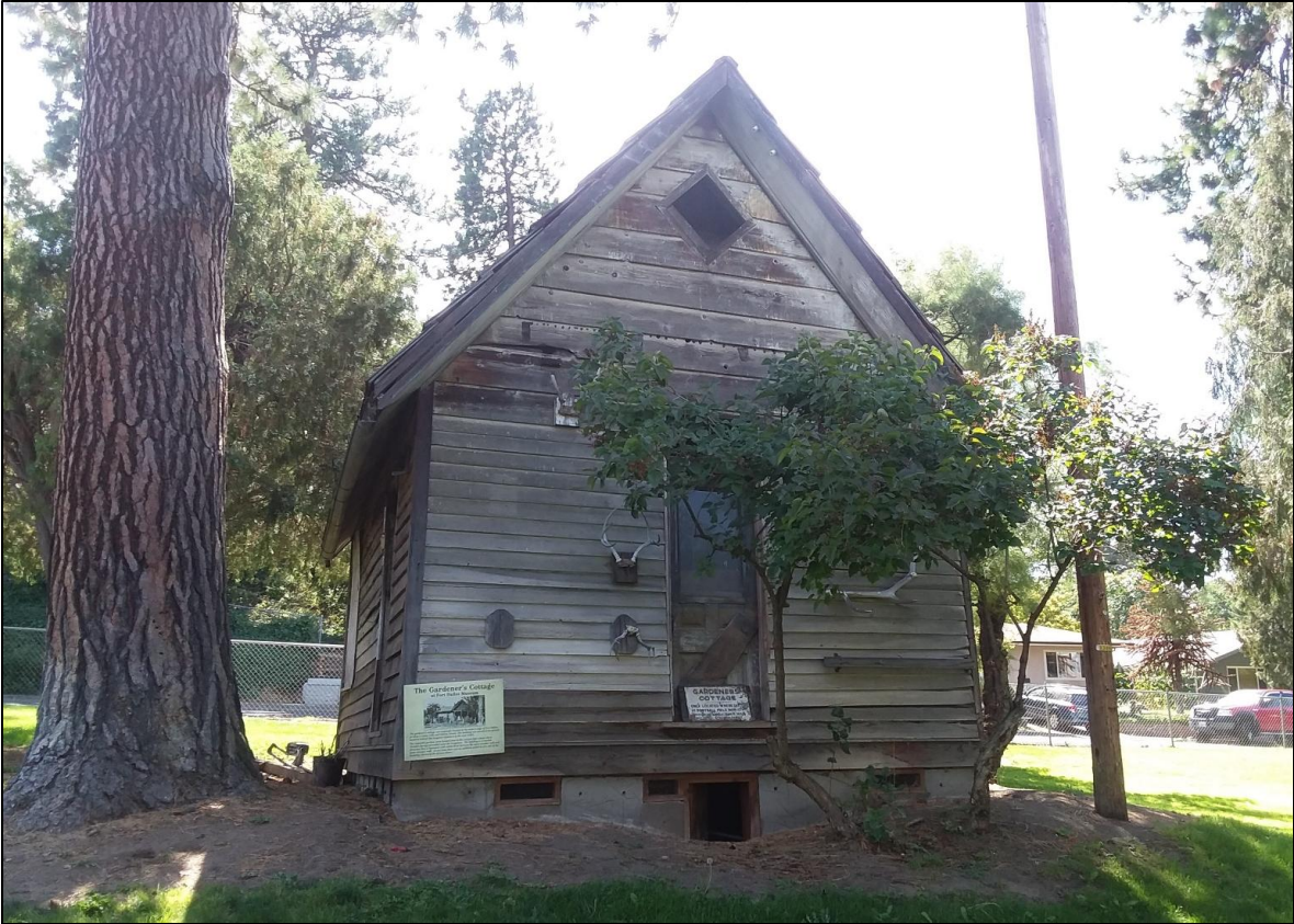
FIGURE 3: NORTHERN WALL OF THE GARDENER'S COTTAGE, FORT DALLES MUSEUM.
