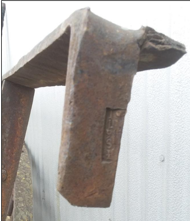
FIGURE 3. MOUNTING PROJECTIONS FROM THE GUARDHOUSE BARS. LEFT IMAGES SHOWS THE STAMP.
