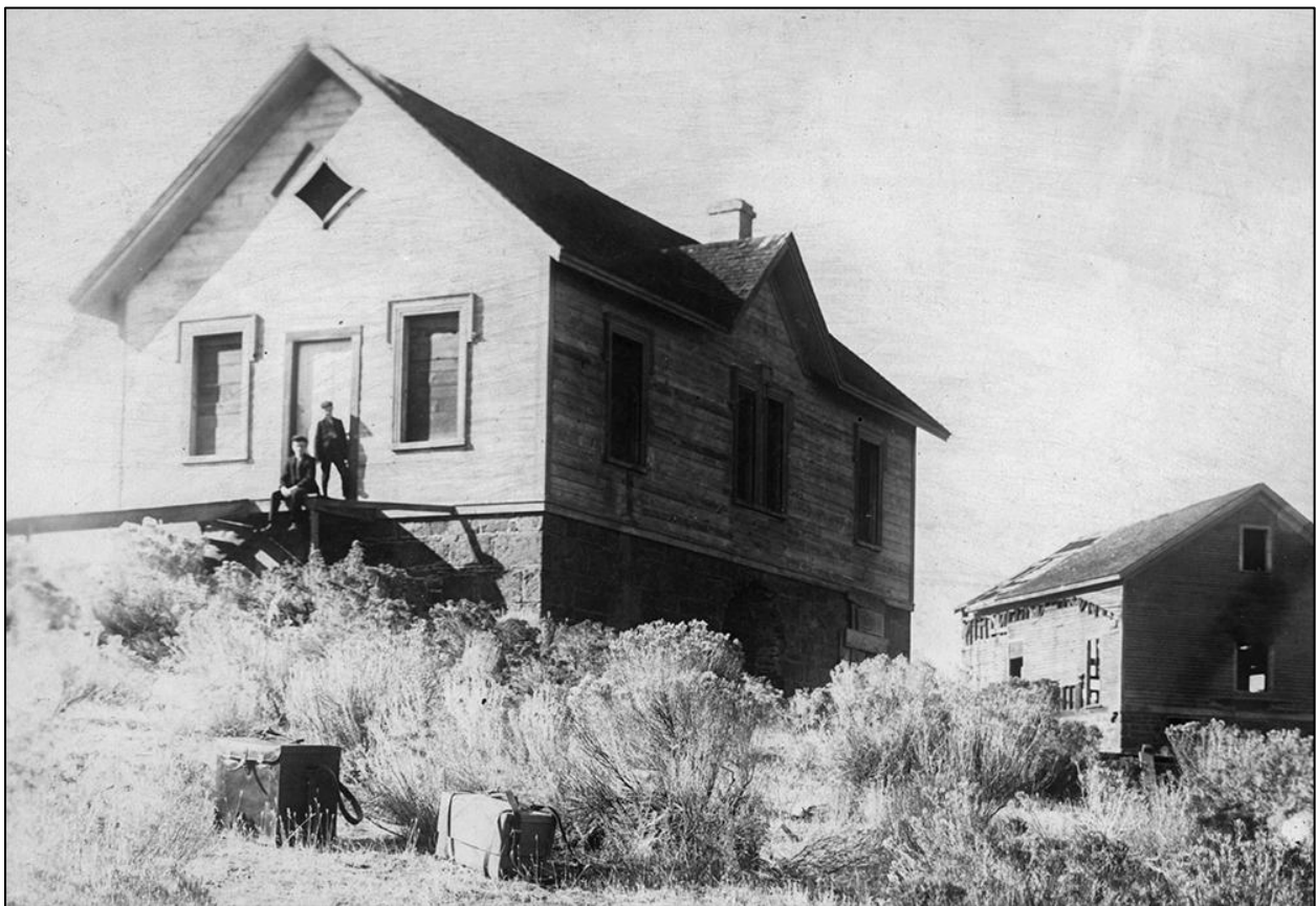
FIGURE 1. ABANDONED GUARDHOUSE, FROM THE OREGON ENCYCLOPEDIA.
